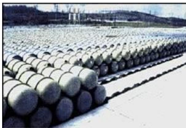
Figure 16. Concrete-floor storage yard for depleted uranium UF<sub>6</sub> cylinders at the Portsmouth, Ohio enrichment plant.
